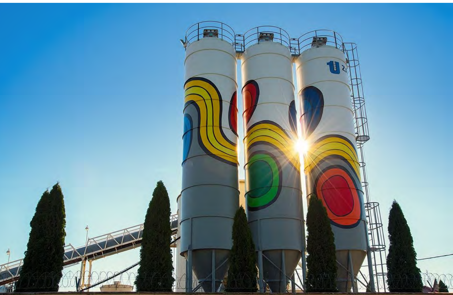
Ready mix-batch plant, Hlohovec, Slovakia
